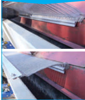
Standing Lock Metal Seam
